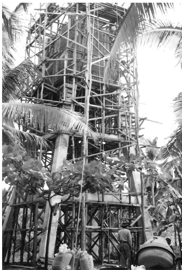
Water tank construction in Cabangahan, San Miguel, Bohol
