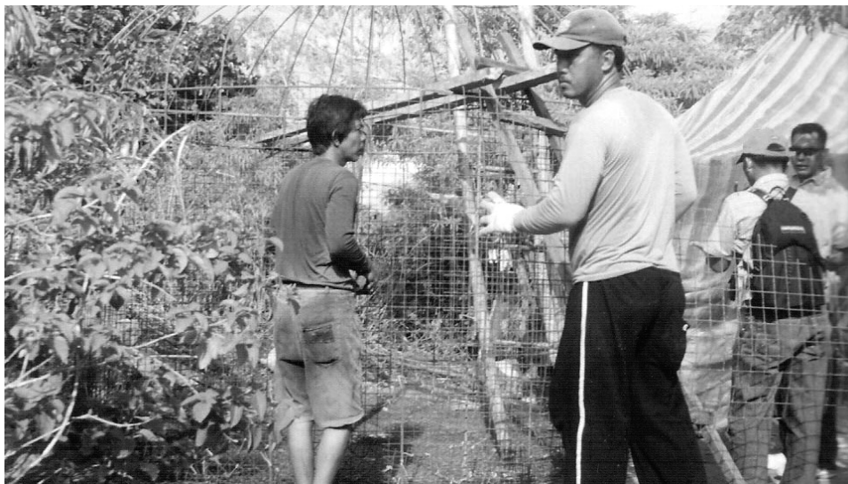
Construction of a ferrocement tank in Maniwaya, Marinduque, a PEF-funded project.
