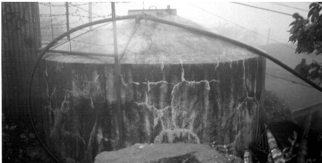
Ferrocement Tank in Irisan, Baguio City
